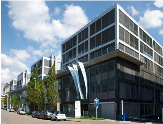
The DBE headquarters in Allschwil (Picture: M. Geering)
